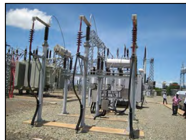
Kiyungi S/S (Reinforcement)
