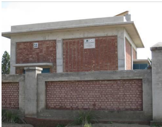
Tubewell Pumping Station (No.11)
