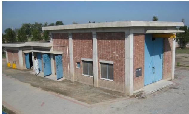
Chlorinator Building at Booster Pumping Station
