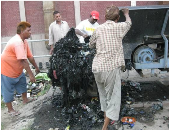
Sanitary Workers Removing Solid Waste from Automatic Trash Rake System
