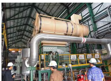
Geothermal Turbine (above) and Generator (below)
