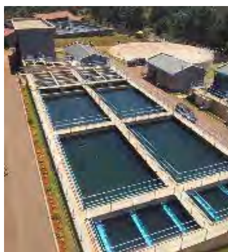
Mukangu Water Treatment Plant Constructed by the Project
