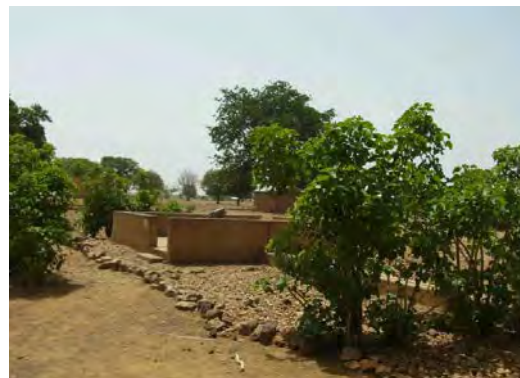
Gravel around the well to avoid a mud puddle and scouring, and hedge to avoid livestock animals (developed by the residents)
