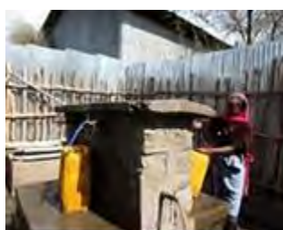
Piped water facility public water faucets
