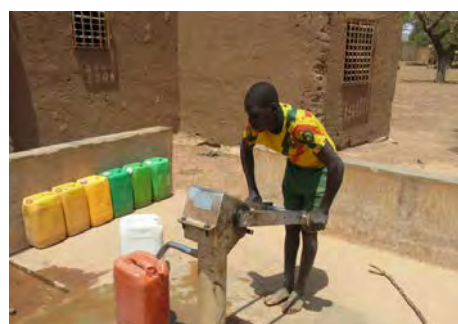
Constructed Deep Well with Hand-pump Facility
