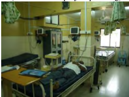
ICU (At the time of project planning)
