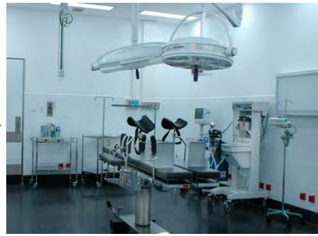
Operating theater (At the time of project completion)
