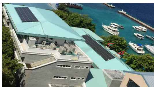
Solar PV Panels on the President Office
