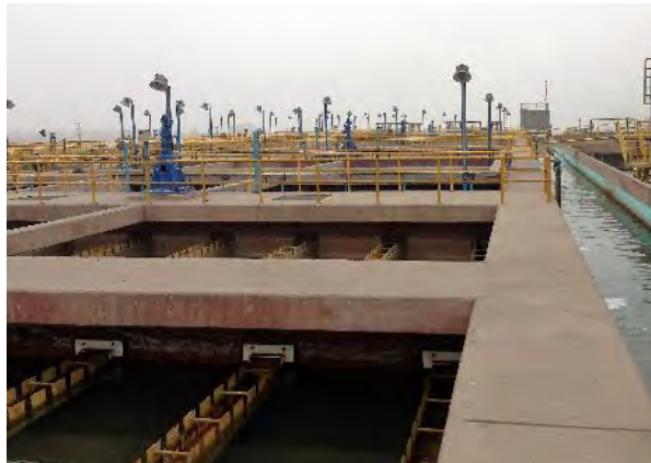
Huachipa Water Treatment Plant
