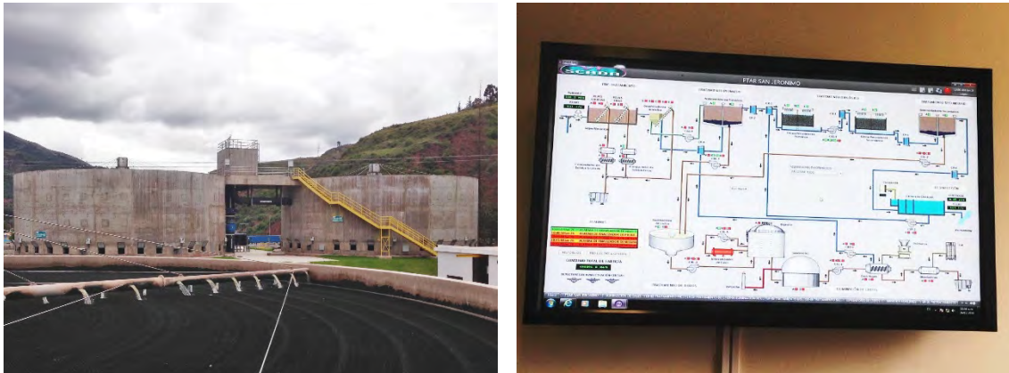
Waste Water Treatment Plant (left) and SCADA system for the Waste Water Treatment Plant (right) in Cusco
