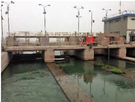
Intake Facility for the Huachipa WTP
