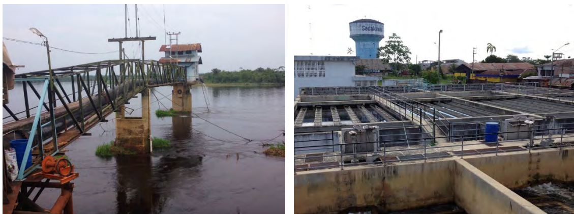
Water intake (left) and treatment plant (right) in Iquitos
