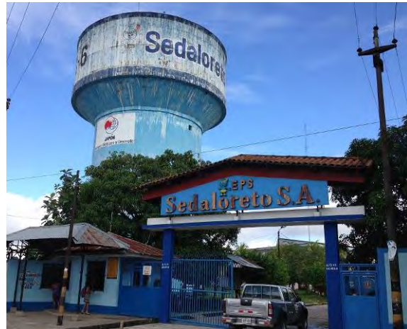
Distribution reservoir constructed at the Iquitos Sanitation Service Company
