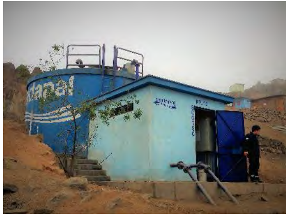
Distribution Reservoir constructed by the Project
