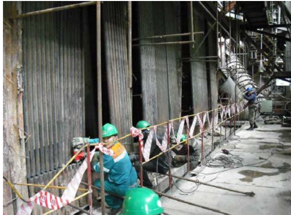
Fig.4.2-27 Replacement of Boiler Water Wall
