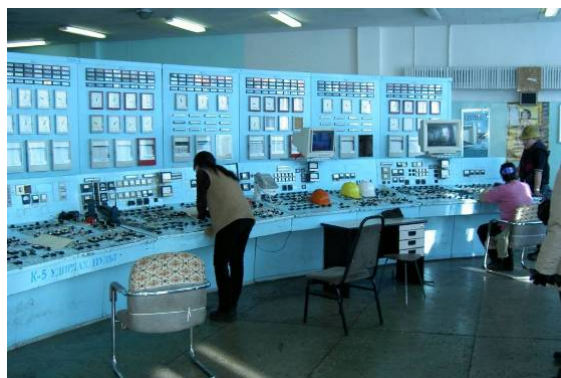
Fig.4.2-18 Boiler Control System before Modification
