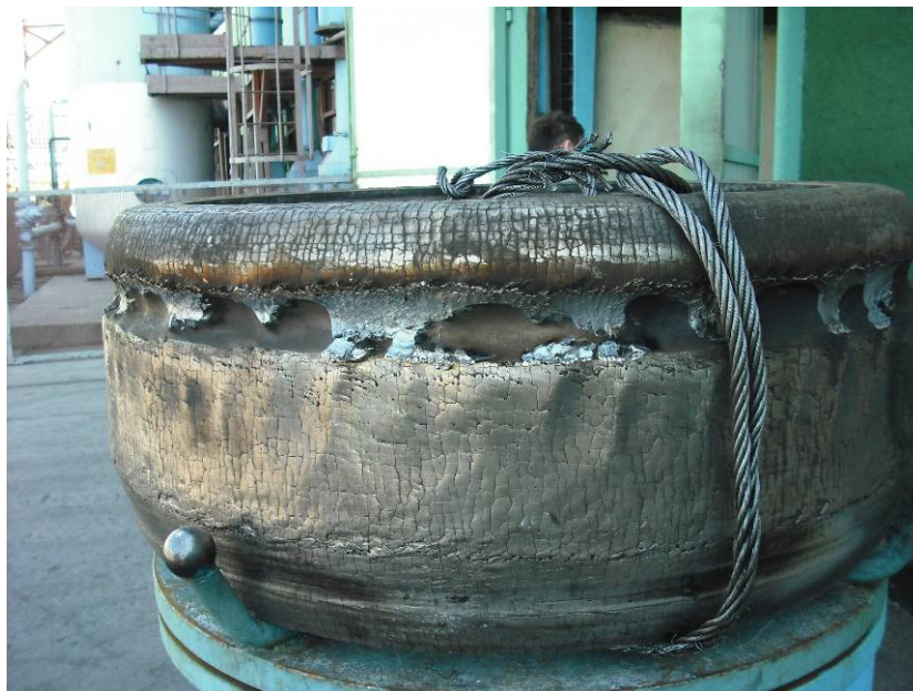
Fig.4.2-11 Mill Roller before Maintenance
