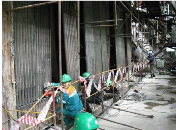
Fig.4.2-27 Replacement of Boiler Water Wall
