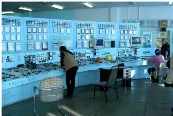
Fig.4.2-18 Boiler Control System before Modification
