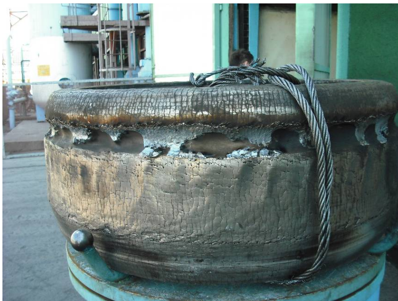
Fig.4.2-11 Mill Roller before Maintenance
