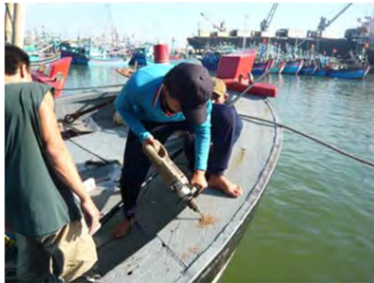
Figure 2-4 Installation of TSS
