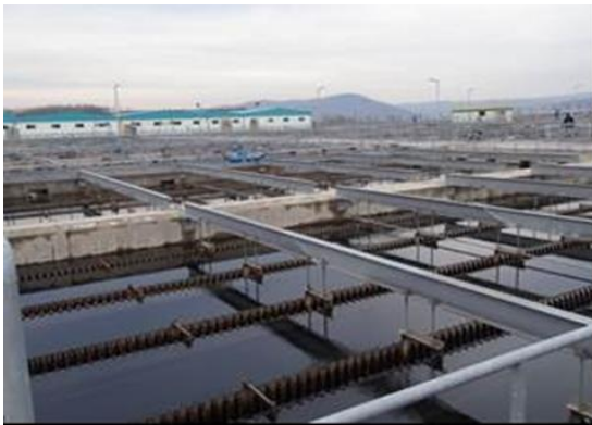
Cumhuriyet Water Treatment Plant
