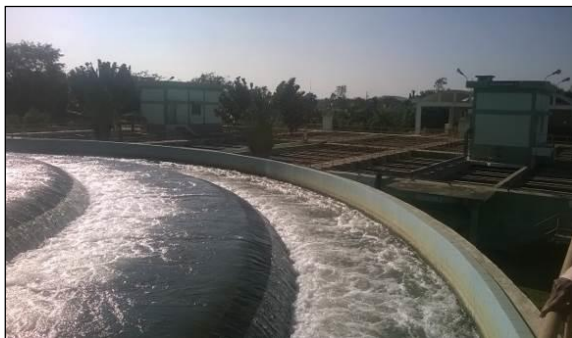
Water Treatment Facility (T.K. Halli)
