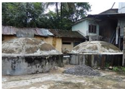
Waste water treatment facility installed at a rice mill utilizing the sub-loan from this project
