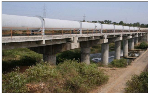
Water Transmission Line to Bangalore City
