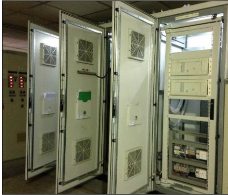
RTU installed (Rawat substation)
