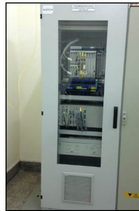
Telecommunication system installed (Substation in Islamabad University)
