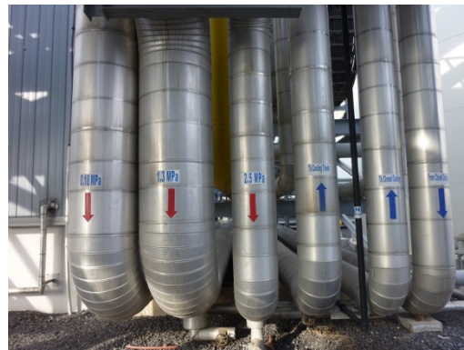
Photo 4: Heat Supplying Pipe
