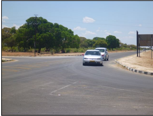
Upgraded Section near Rundu
