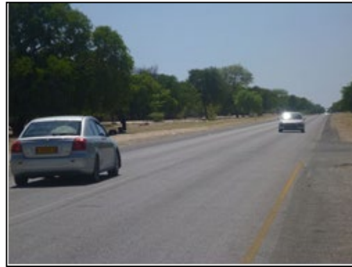
The road improved by this project
