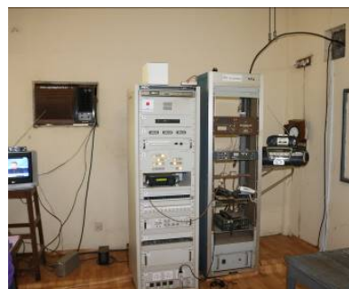
Program input equipment rack
