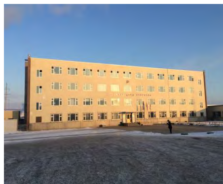
A school constructed by the project (No.118 school)
