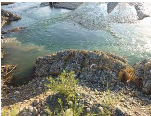
Photo 3: Gabion Fell Down due to Typhoon Koppu of 2015 (Region I: Ilocos Norte)
