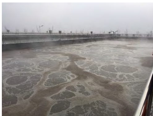
A biological reaction tank at a sewage treatment plant
