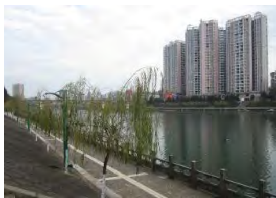
Dike Constructed (in Chibi City)
