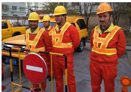
A water pipe maintenance and inspection team
