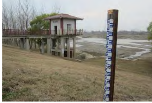
Dike and culvert gate (Xiaogan City)
