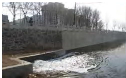
Water treated at the Gongzhufu sewage treatment plant and discharged to a branch of the Xiaohei River
