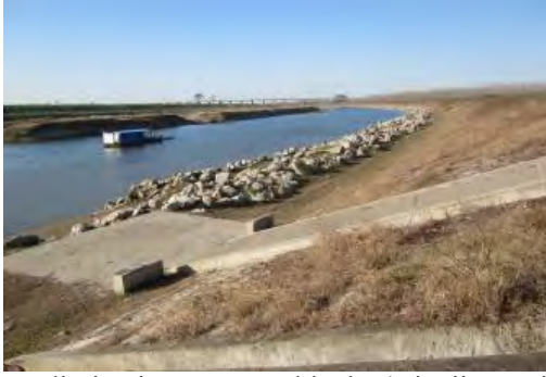
Wave-dissipating concrete blocks (Qianjiang City)
