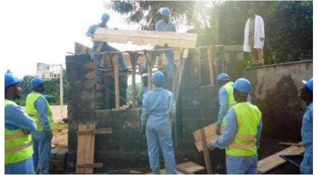
Guard house construction
