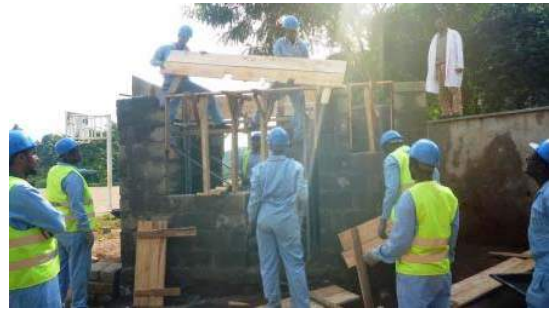
Building Construction Training at KTTC (Guard house construction practice)
