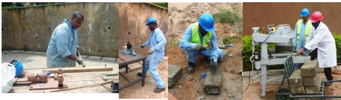
Bending a steel frame with (right) and without (left) a machine
