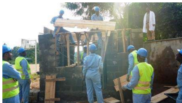
Guard house construction
