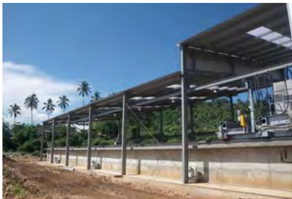
Air blowers installed at the sidewall of primary fermenter
