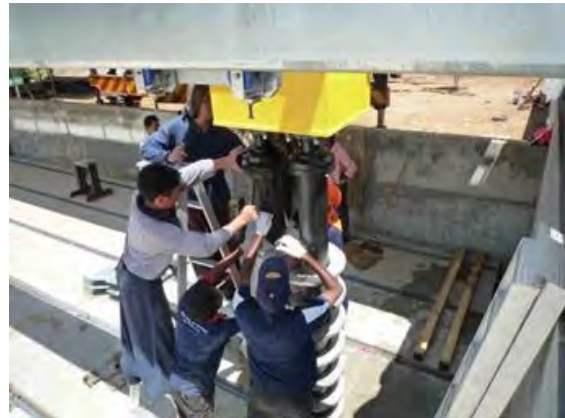
Picture 5 RA-X assembly work
