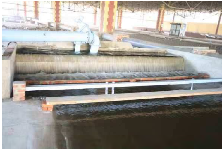
Photo (4): Model Entrance after Construction
