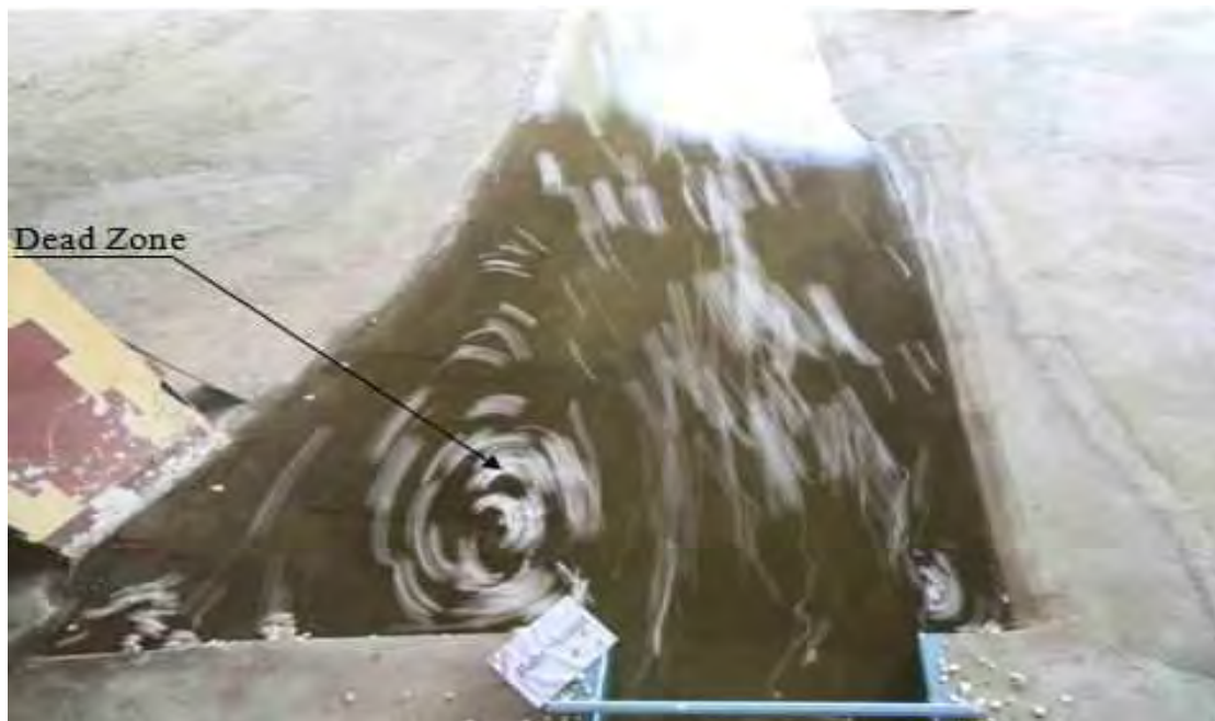
Figure (15): Formation of Dead Zone Downstream Bahr Yusef New Regulator
