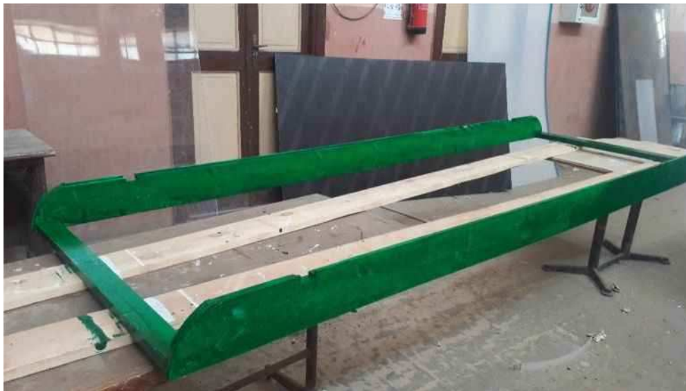
Plate (1A) Manufacturing of the Half Pier
