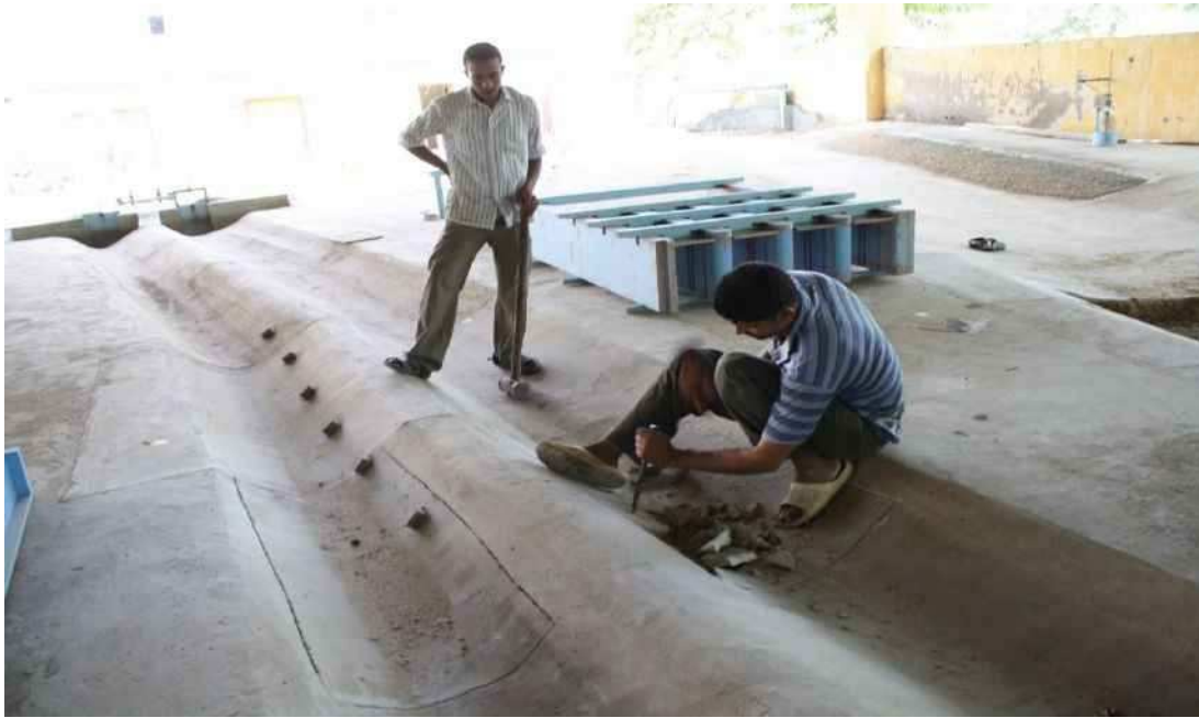
Figure (7): Physical Model Preparation to Place the New Regulator
