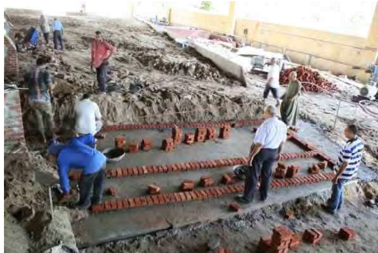
Photo (3): Model Entrance Construction
