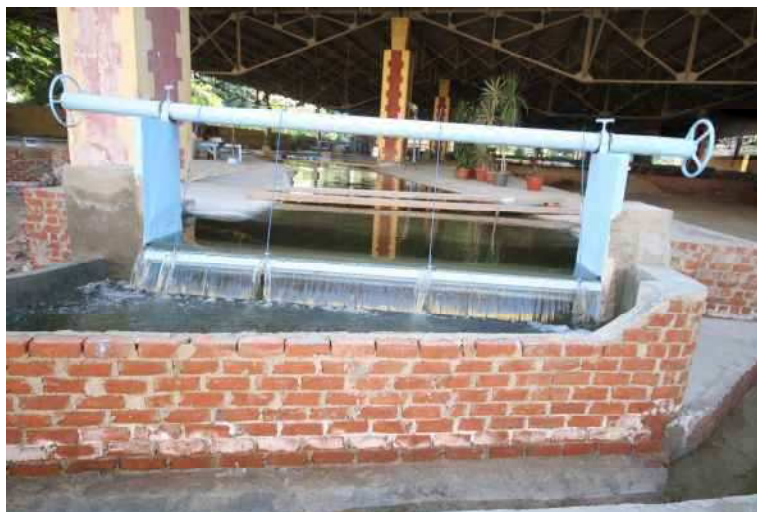
Photo (7): Sharp Crested Weirs of Badraman and Daytutiah Canals
