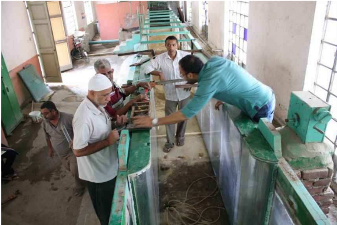
Plate (4A) The Model During the Construction Inside the Flume
