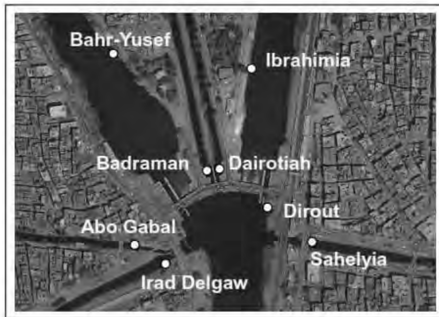
Photo (10): layout of the Existing Dairut Group of Regulators
