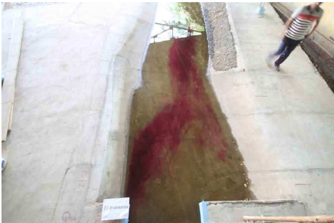
Photo 14: Flow Tracking Downstream New Ibrahimia Regulator Using Colored Dye
