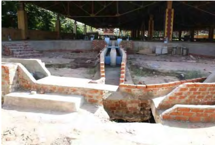
Photo (7): Sharp Crested Weirs of Badraman and Daytutiah Canals
