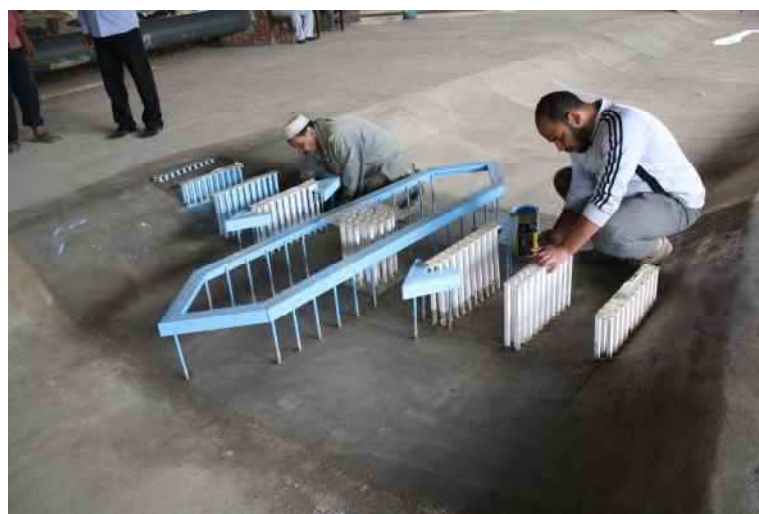
Photo (19): El-Korashia Bridge Construction
