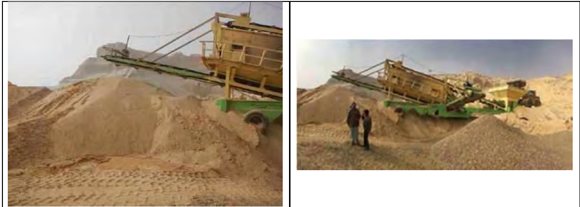
Figure 1-4 Sand and Screening Machine
