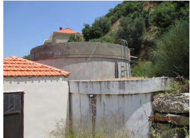
配水池(奥400m 3 +手前50m 3 程度) Aamatour in Aley District
