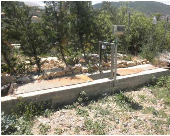
Jdeidet El Chouf Municipality in Alay District の下水処理場流入渠 (2016.6.18)
