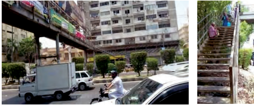
Photo Pedestrian Bridge on the Sharee faisal road
