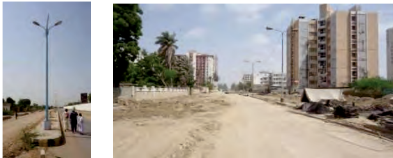
Photo (Left) Example on Access road to the N5, (Right) New construction in the Karachi City
