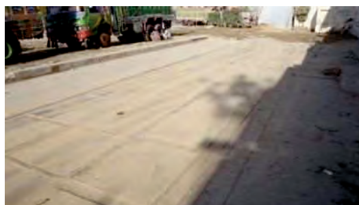
Photo Existing Weight Bridge
