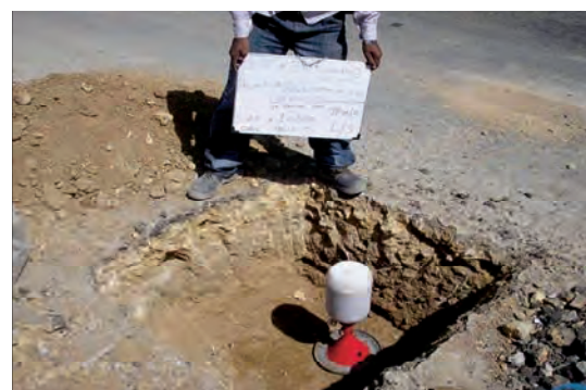
Photo-2 Field density test
