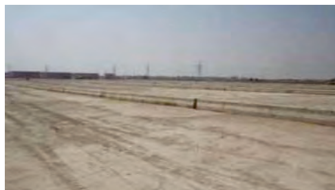
Photo Tank Lorry Parking Area under Construction
