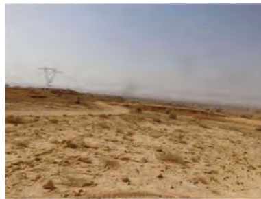
Photo Nooriabad (Subbase course)
