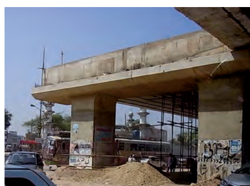
Photo F/O construction site in the east side (under construction)
