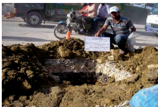
Photo-1 Trial pit sampling
