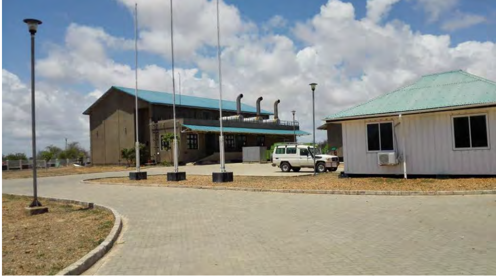
Existing TANESCO 8MW gas fired generators at SomangaFungu Site.
