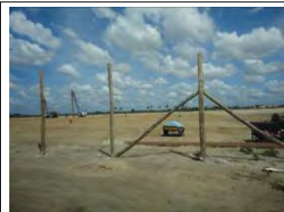
Site View (Piling)
