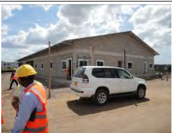
Office (Under construction)
