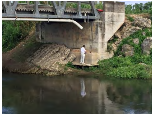
Measurement for Rebound Number on Right Abutment
