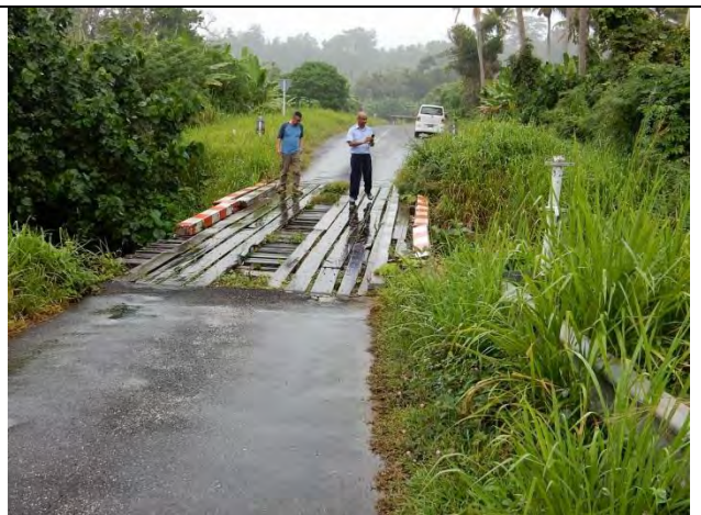
Aging Bridge (Lamin Bridge)
