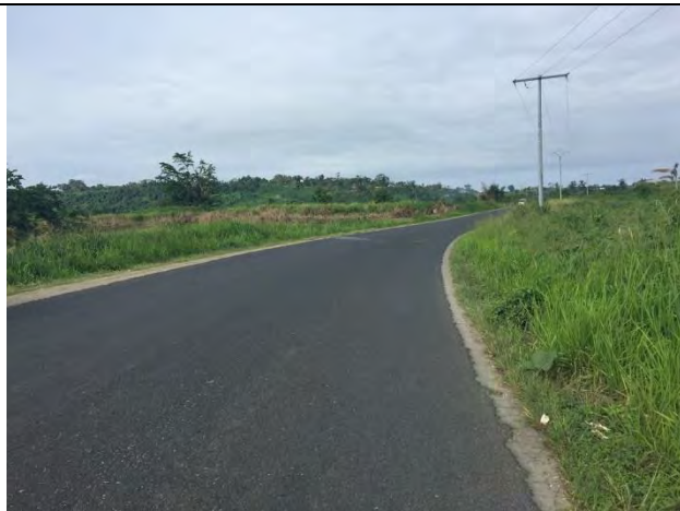
Road Improvement Site
