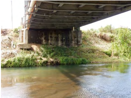
Damage on Gabion Protection (Left Bank)
