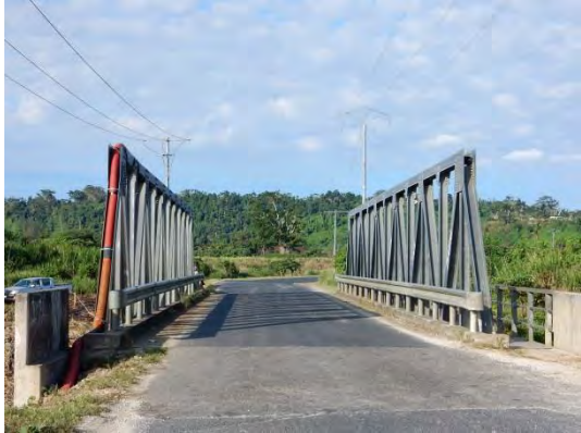
Superstructure (good condition)
