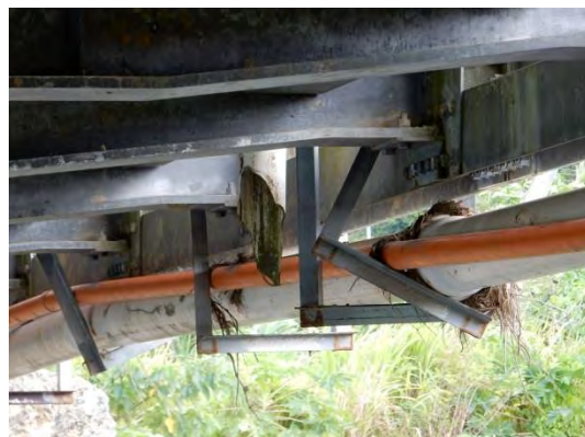
Damage on Drainage Pipe
