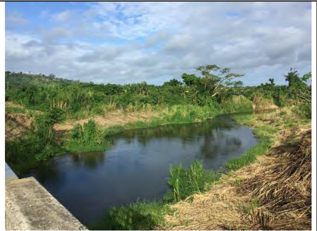
Slope Protection Site (Downstream, Left Side)
