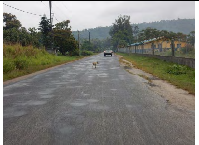
Ring Road Condition (South of Efate Island, around Mele)
