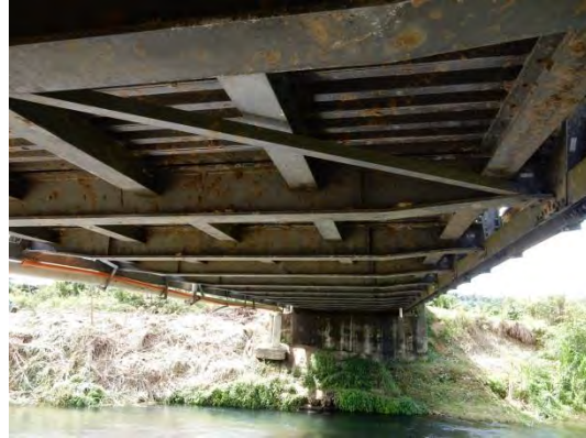
Superstructure (good condition)
