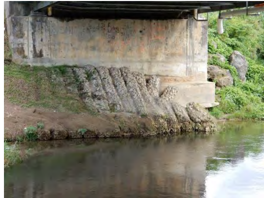
Damage on Gabion Protection (Right Bank)
