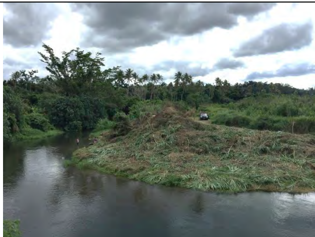
River Condition (Upstream of Teouma Bridge)
