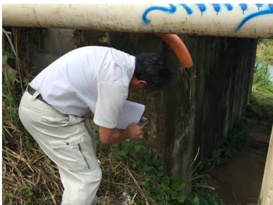
Measurement for Rebound Number on Left Abutment
