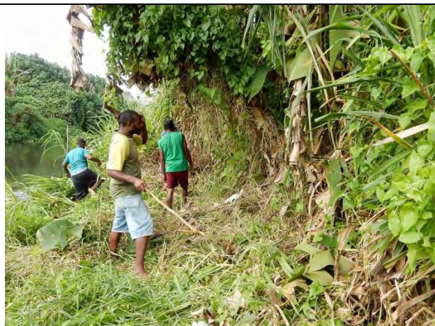
Vegetation along River (Upstream, Left Side at around St. 4900, under Cutting)
