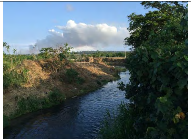
River Widening Site (Upstream, Left Side)
