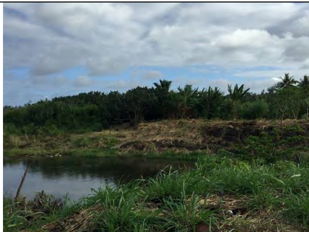
Slope Protection Site (Downstream, Right Side)
