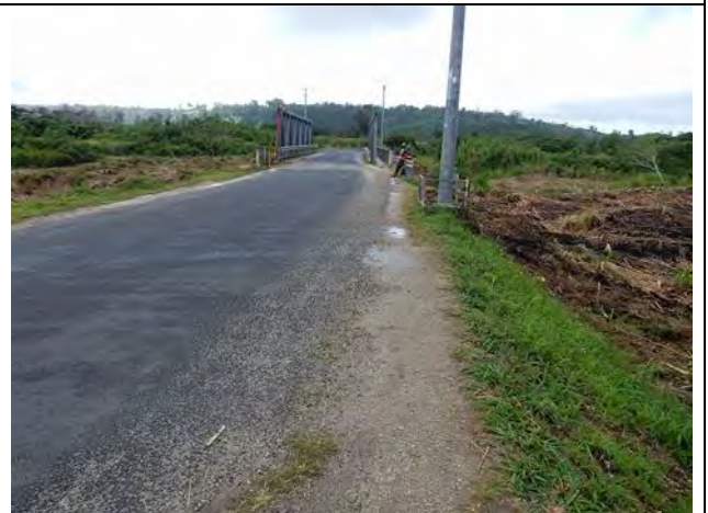
Left Approach Road at Teouma Bridge (Bridge Rehabilitation Area)
