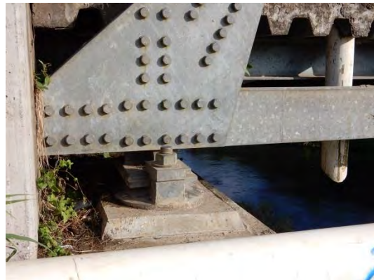
Hinged Bearing (good condition)
