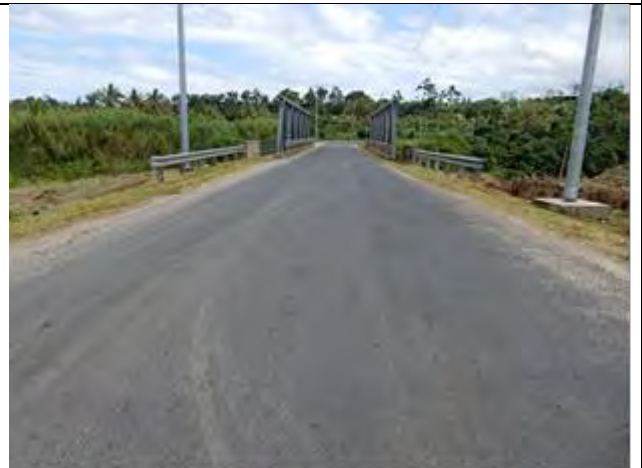
Present Road Condition Improved in "the Project For Rehabilitation of Bridges on the Ring Road in Efate Island"
