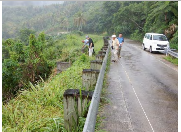
Klems Hill Slope Failure Area
