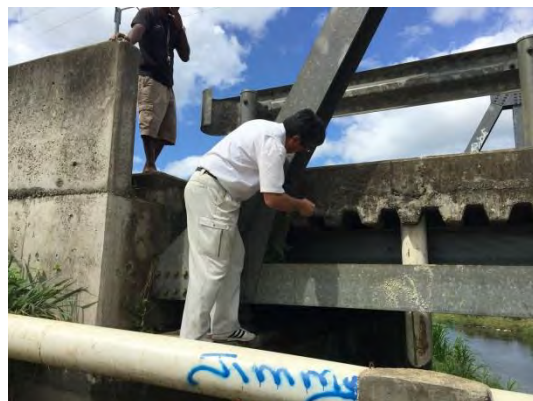
Measurement for Rebound Number on Concrete Deck Slab
