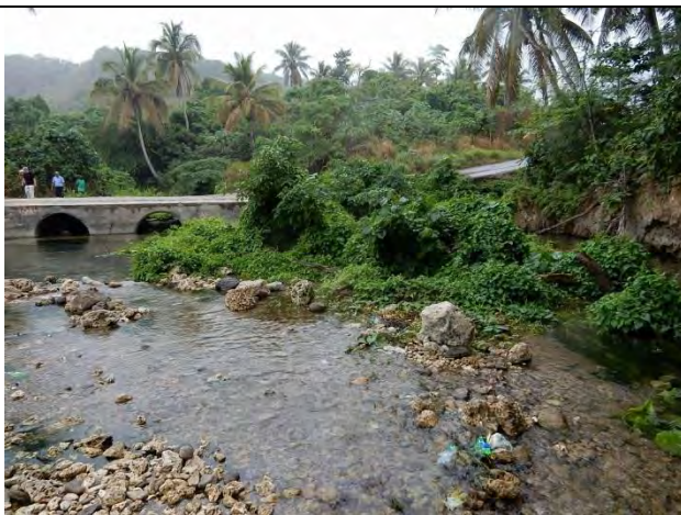
Sedimentation and Trees Blocking Cross Section Area in River (Creek Ai Culvert)
