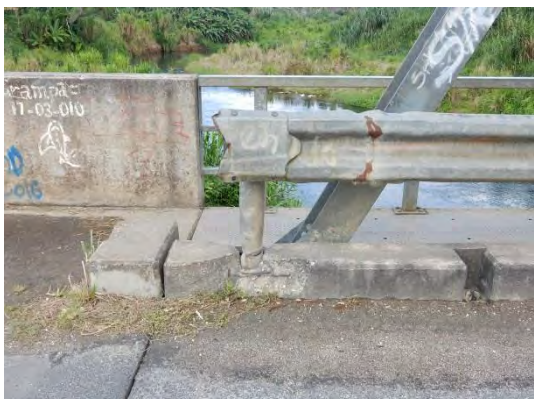
Damage on Railing and Curb
