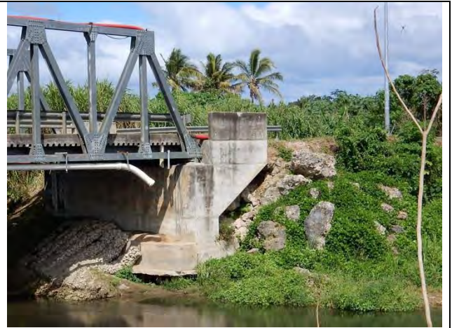
Urgently Rehabilitated Approach Road
