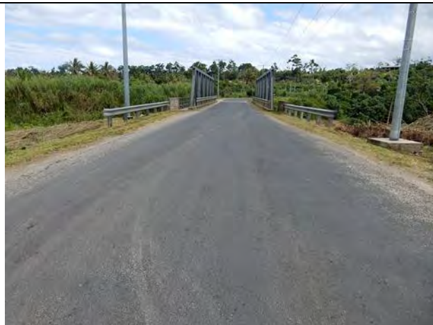
Right Approach Road at Teouma Bridge
