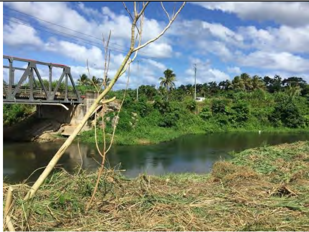
Slope Protection Site (Upstream, Right Side)
