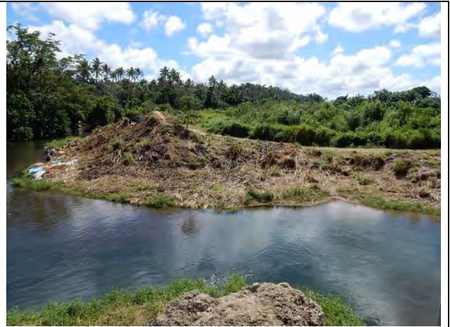
Sedimentation inside of Curve (Upstream, Left Side)
