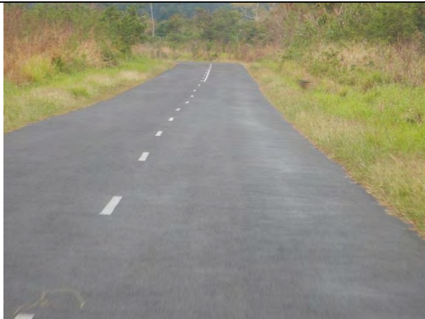
Ring Road Condition (North of Efate Island, around Port Havannah)
