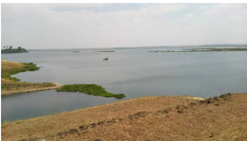
Reservoir of North Nawin Irrigation System
