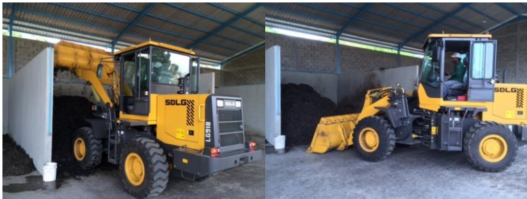
Figure 5 Wheel loader mixing and stirring the organic waste
