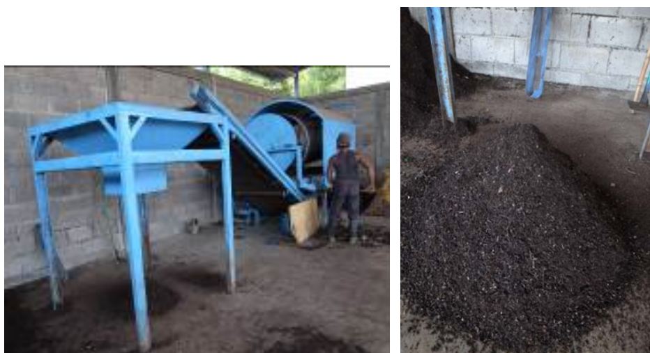
Figure 10 Left : Trommel screen, Right : Compost (final output)
