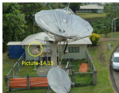
Picture 13: Cable Ladder Location
