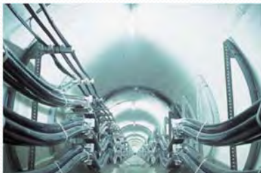
Underground power line construction work management
