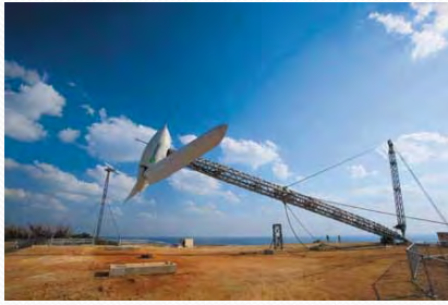
Structural reengineering of foreign-made WT tower to ensure compliance with Japanese standard
