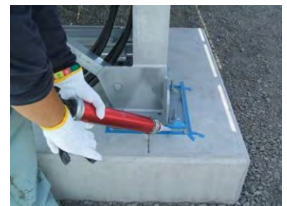
Caulking the contact surface between the rack and foundation
