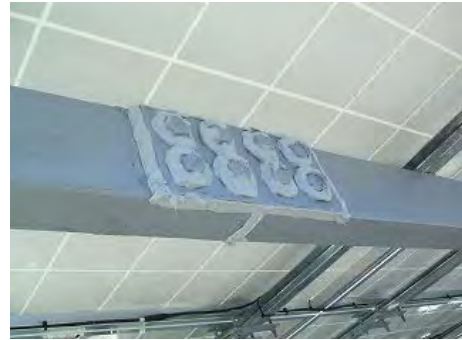
Bolt joints being caulked
