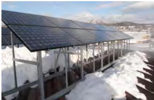
Figure 3.2-4: Installation of PV array in heavy snow area
