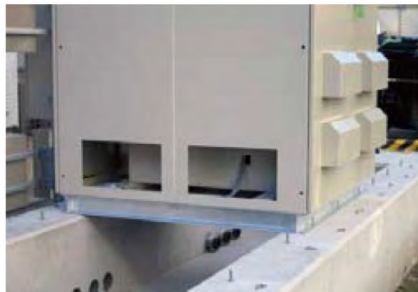
Foundation work for PCS
