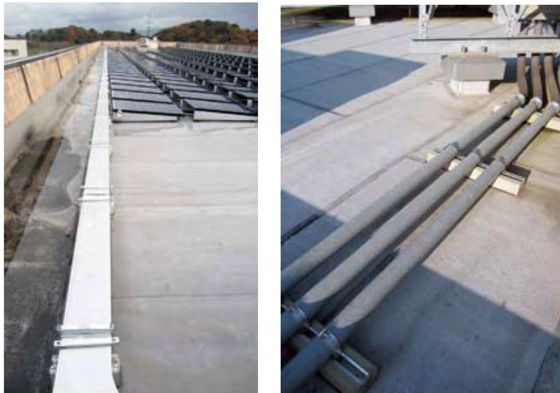
Figure 3-9: Cable installation between PV array and junction box
