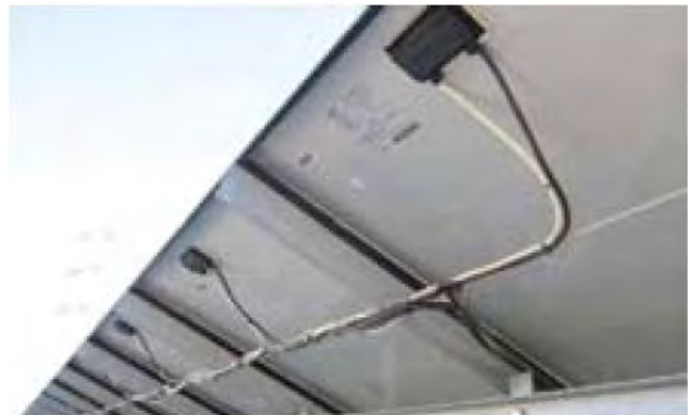
Installation with messenger wire
