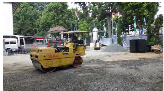
Backfilling Work (Sep.-6,2015)
