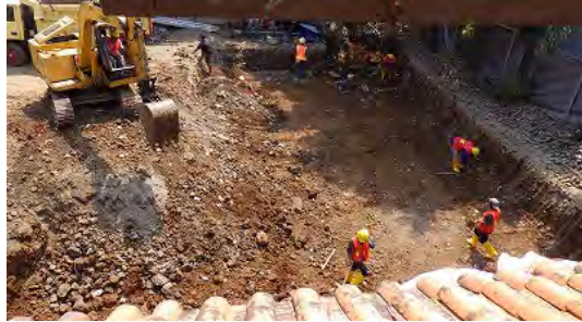
Excavation Work (Aug.-27,2015)
