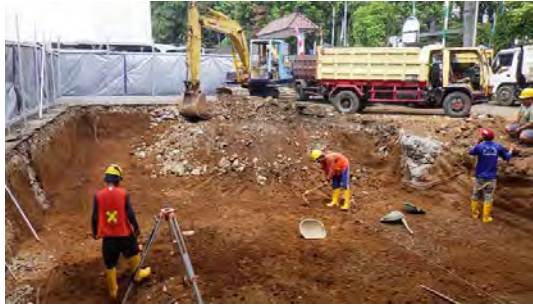
Excavation Work (Aug.-30,2015)
