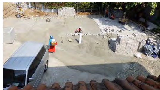
Concrete Block Pavement Work (Sep.-13,2015)
