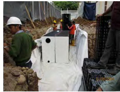
Building Work of New Trench-kun (Sep.-1,2015)
