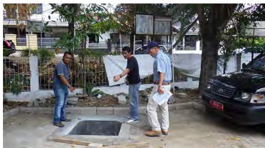
Site Inspection by Bogor Staff (Sep.-26,2015)
