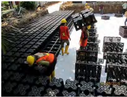
Building Work of Pladam-kun (Sep.-1,2015)
