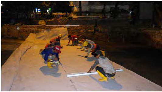
Sheet Laying Work (Sep.-1,2015)
