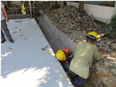
Setting Work of Root Barrier Sheet (Sep.-2,2015)
