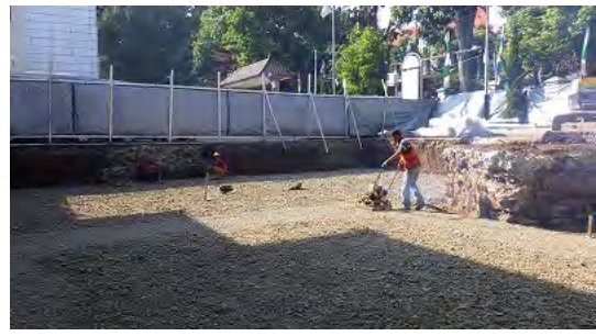
Foundation Work (Sep.-1,2015)
