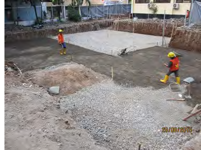
Foundation Work (Aug.-29,2015)
