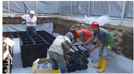
Building Work of Pladam-kun (Sep.-2,2015)
