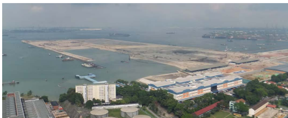
Figure 2.4.43: Reclamation of Pasir Panjang Phase 3 & 4 in Progress
