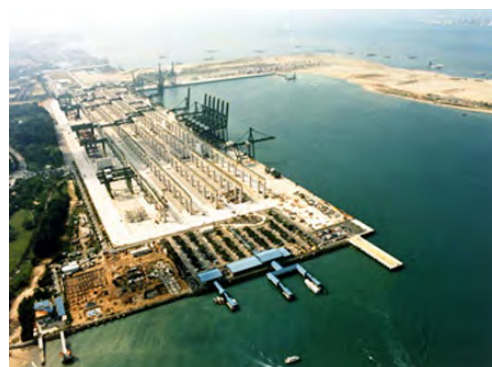
Pasir Panjang Terminal under construction Source: Penta-Ocean Construction co., ltd ( http://www.penta-ocean.co.jp/english/project/facility/harbor/012.html )
