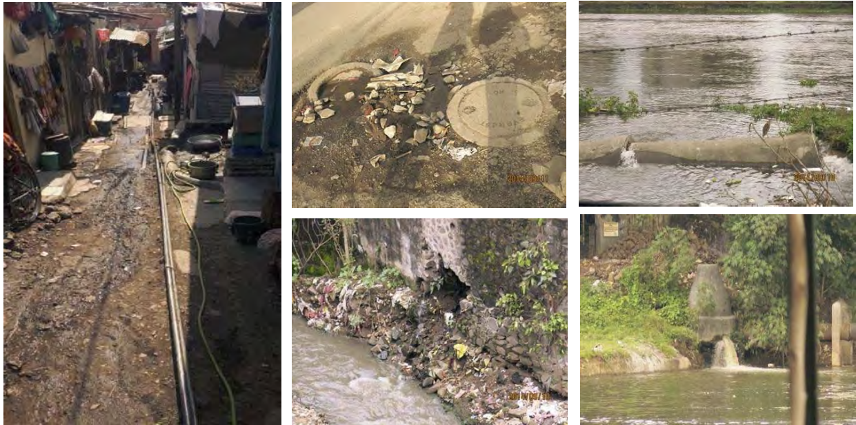
Sewage flowing in Slum area
