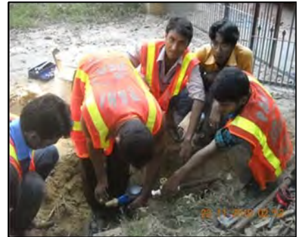
The CWASA staff replacing meters, with uniform work clothes labelled "PANI-1".
