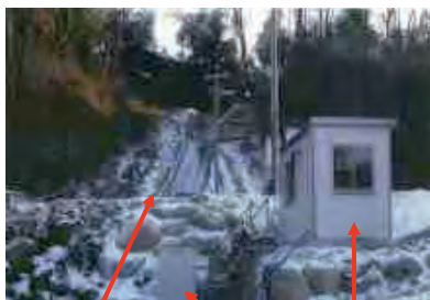
Komagane natural-energy-based small hydroelectric power plant No. 1
