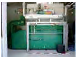
Wooden chip boiler
