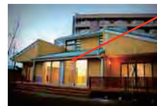
Appearance of daycare center of Asama General Hospital
