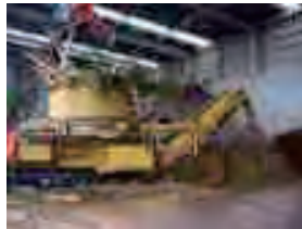
Crushing and chipping timber offcuts
