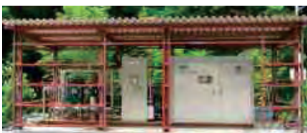
Binary power generation facility at Shichimi onsen hotel
