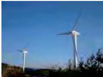
Hokigamine wind power plant (Tosayamada town, Kami city)
