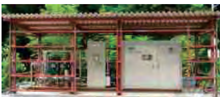
Binary power generation facility at Shichimi onsen hotel
