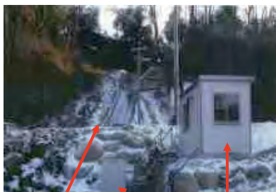
Komagane natural-energy-based small hydroelectric power plant No. 1
