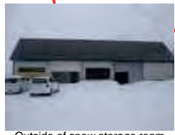
Outside of snow storage room (renovated old JA storage house)
