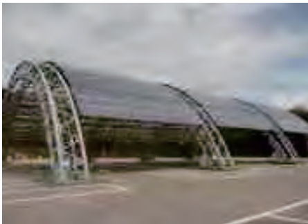
Solar PV system (Noichi animal park)
