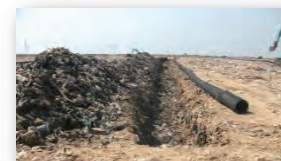
Installation of gas collection pipes
