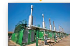
Electricity generated using GE 320 1063 KW biogas engines
