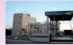
Fuel-production facility for used cooking oil in Kyoto (Produces 4,000 liter/ day)
