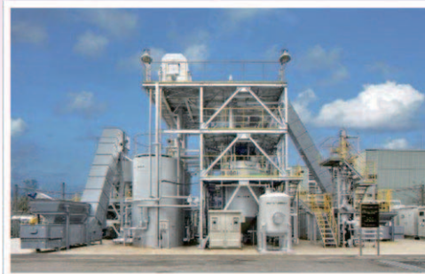
Demonstration plant located in Kyoto (2011)
