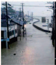
Kumano river overflow due to Typhoon No.12 in 2011 (Kihou town, Minamimuro-gun) (provided by: Ministry of Land, Infrastructure and Transport)
