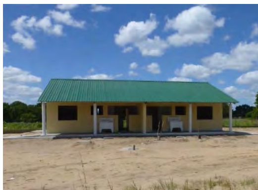
Photo 6: Teachers' house of Manjakaze school (under construction)
