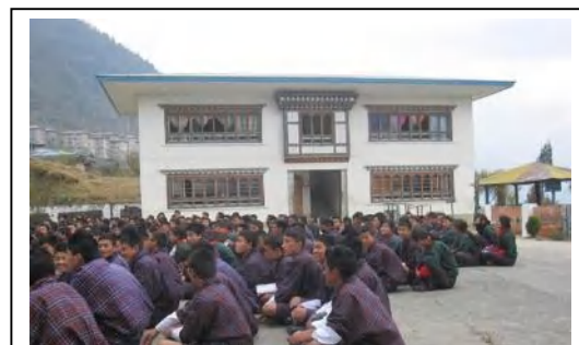
Four-classroom building Chukha School, Chukha District
