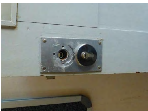
Photo 11: Broken doorknob (Chissano school)
