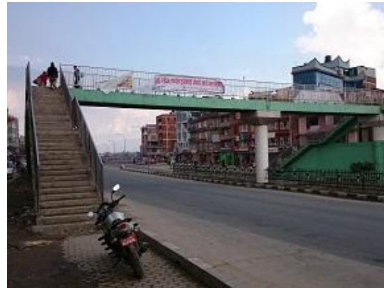
Picture 2 Overhead bridge (Constructed by the Nepali side)
