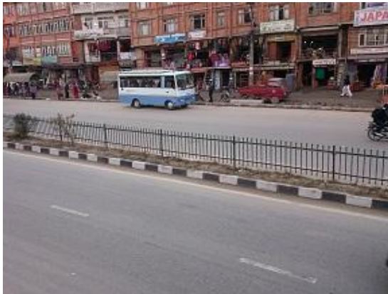
Picture 1 Guard fences at the median strip
