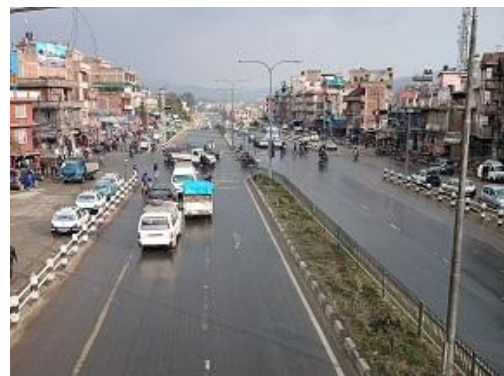
The road developed in this project
