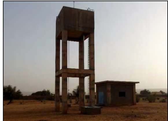
Water Supply Facility Constructed by the Project
