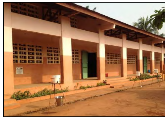
Photo (Right) Solid classrooms constructed by the project
