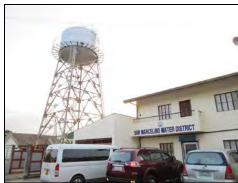
Elevated Water Tank constructed in this Project (San Marcelino Water District)
