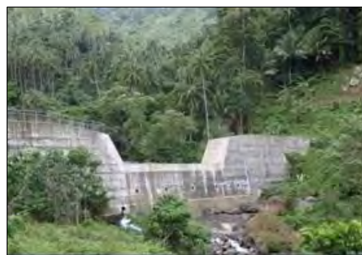
Sabo Dam (Upper Dam)
