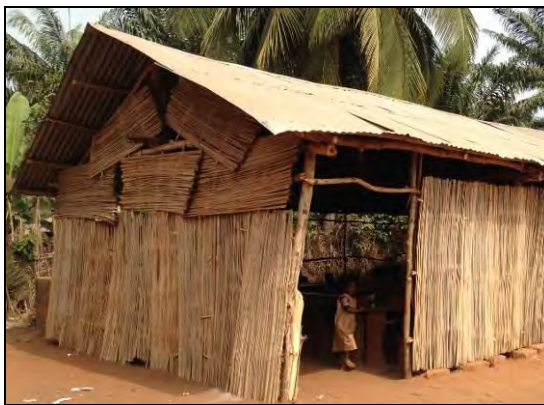
Photo (Left) Simple classroom
