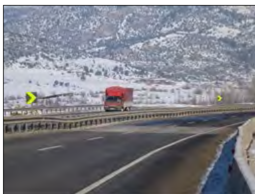
The road section improved by the project
