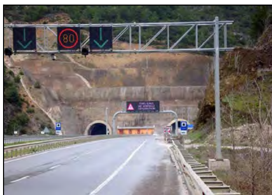
Photo 1: Tunnel of the State Road D650
