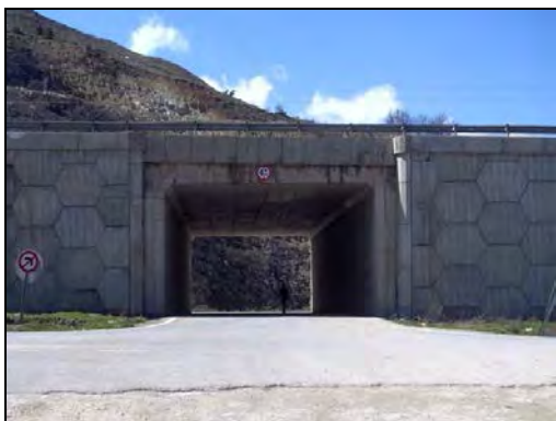
Photo 3: Passage under the State Road D650
