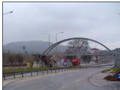
Photo 4: Pedestrian overpass on the State Road D650
