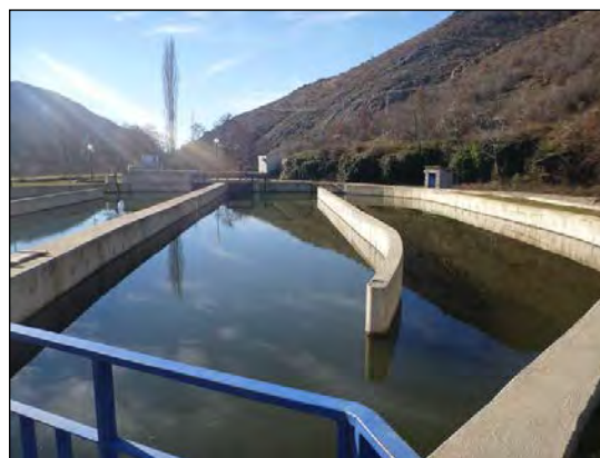
Photo 2: Water Intake No.3
