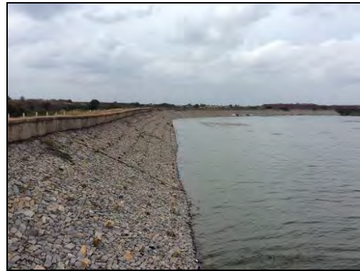
Alaganur Balancing Reservoir constructed under the Project
