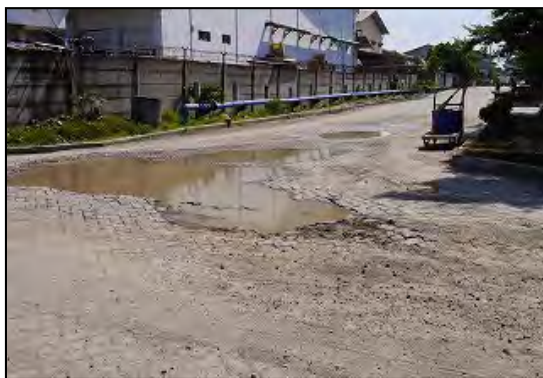
Photo 17: Puddle caused by the broken roads inside of JFP (At the time of the Ex-post Evaluation)
