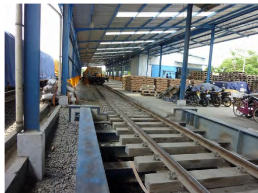
Railroad bed developed by this project (track laid with Indonesian funds)
