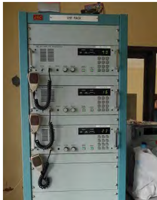
GMDSS (VHS/DSC) Equipment (Kalianget CRS)
