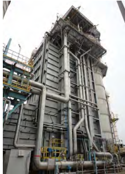
Heat Recovery Steam Generator
