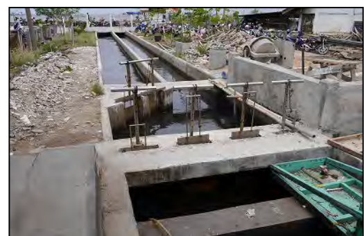
Photo 8: Sea Water Cleaning System (At the time of the Ex-post Evaluation)
