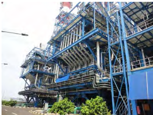
Heat Recovery Steam Generator
