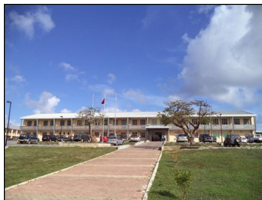
Outpatient Department Building Constructed in the Project
