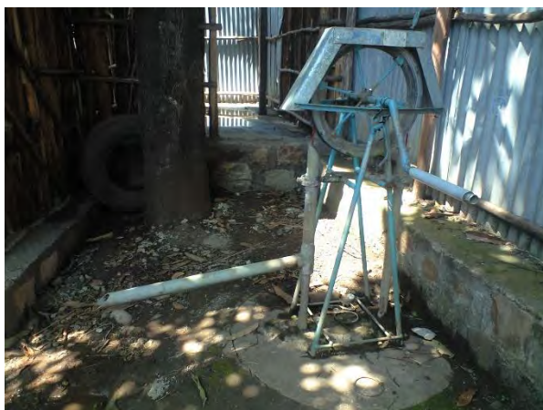
Household rope pump installed in the Project 2
