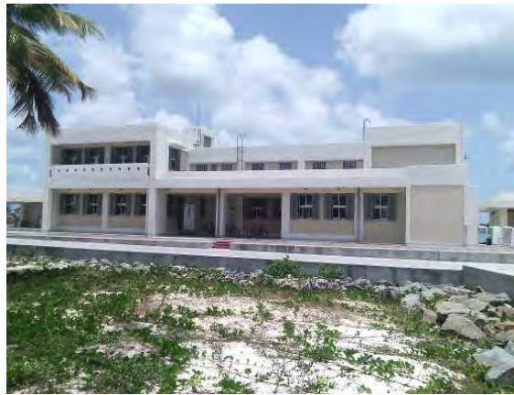
The Fisheries Complex constructed under the Project in Barbuda Island Codrington area
