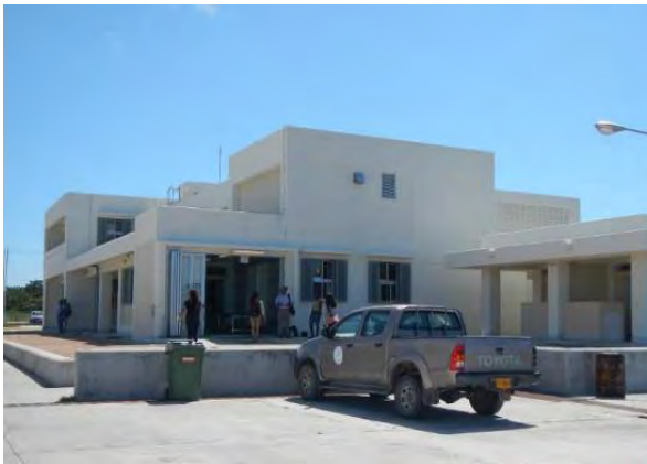
Entrance to the fish handling room of the fisheries facilities (at the time of the ex-post evaluation)
