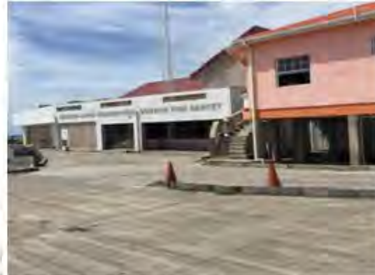
New Fisheries Center after Rehabilitation
