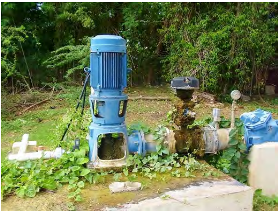
A well without proper cleaning (Cookson 3 Well)
