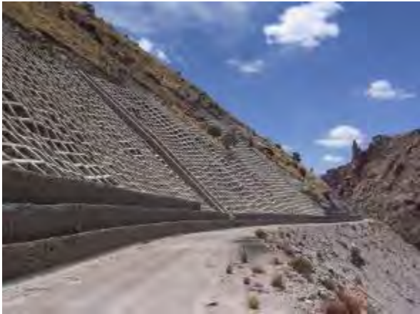
Slope Protection for the Access Road to Water Intake
