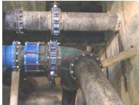
The pipe repaired at the Aranjuez WTP
