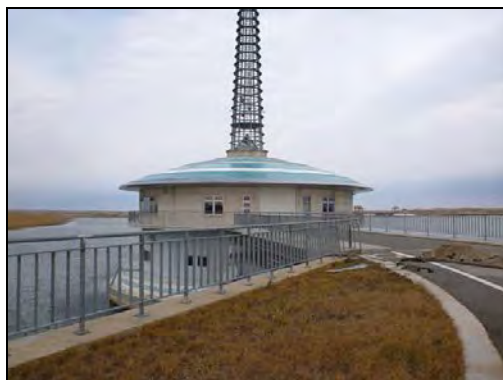
Water Intake Facility Constructed by the Project
