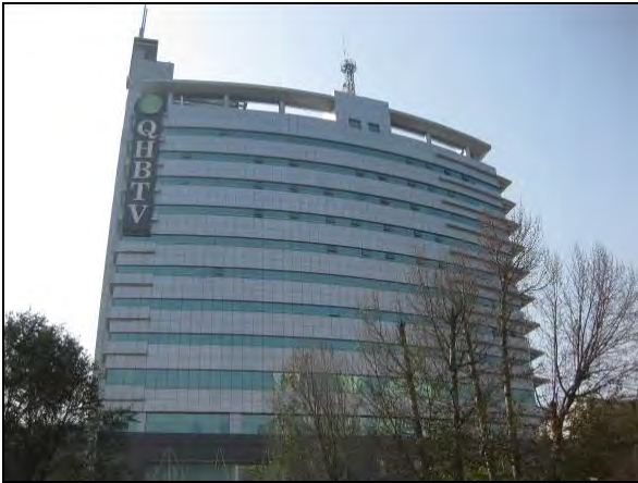
Qinghai Radio and TV Station (QHBT) 1
