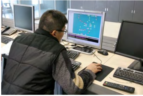
Radio wave monitoring in BMS
